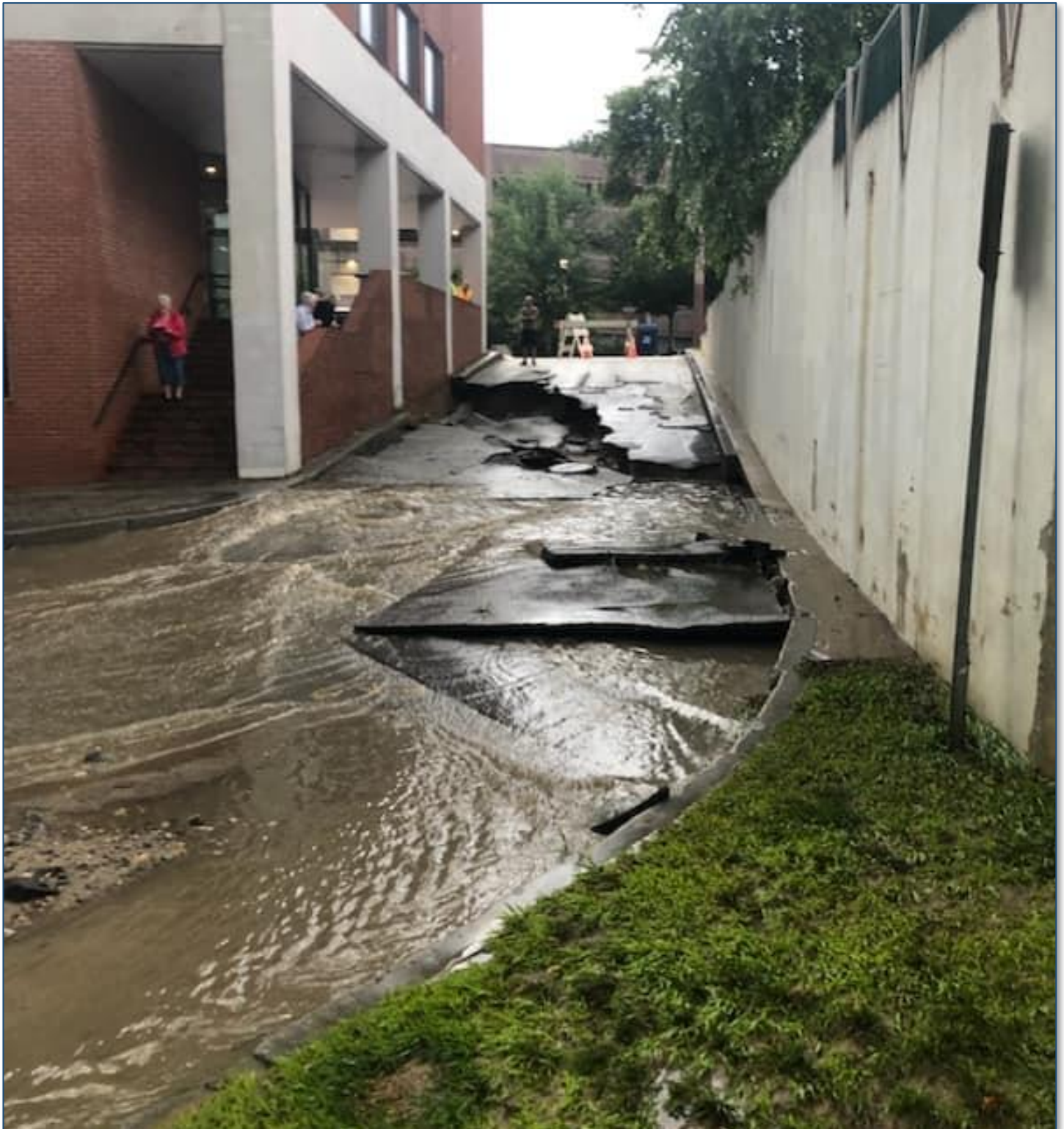
Figure 44: Miller Alley, Auburn, ME July 25, 2023. Source: City of Auburn.
